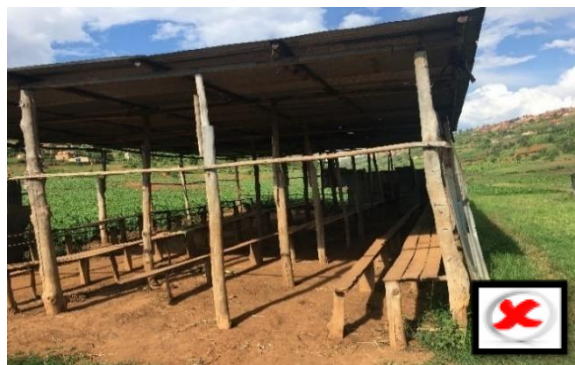
Figure 61 Not ideal grading shade
